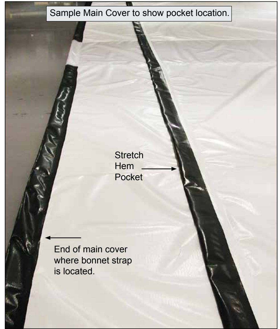
Photo above shows a similar cover and location of stretch pocket. Underside of cover is shown, which is visible from inside building when cover is installed.
